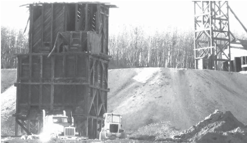
(5) After Structure Has Been Placed and Prior to Wind
