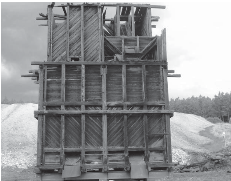
(6) After Stabilizing and Back on Pad
