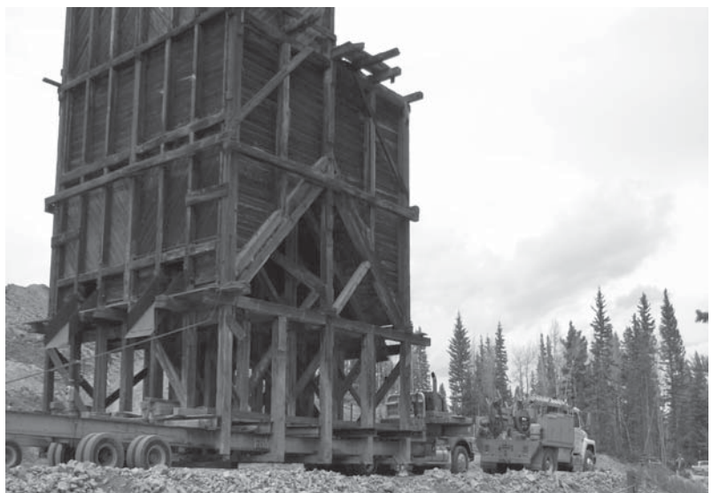
(3) Structure in Process of Moving to New Site
