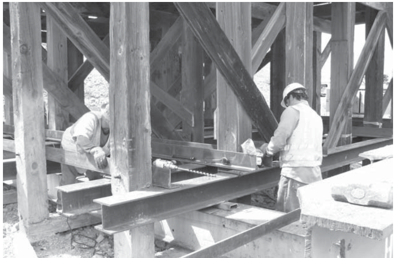
(2) Preparing the Ore House structure for the move.
